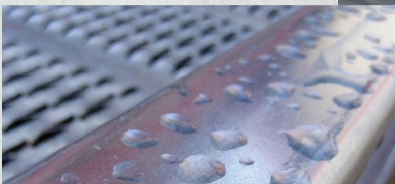
Supporting beams and steps made of hot dip galvanized steel
